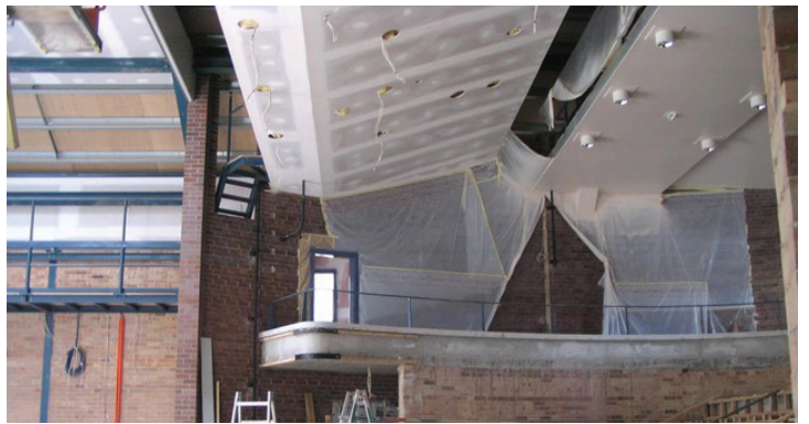
Hoskins Centre theatre under construction
