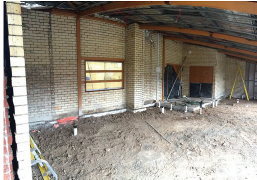
Creating new girls' changeooms in the eastern side of the gym
