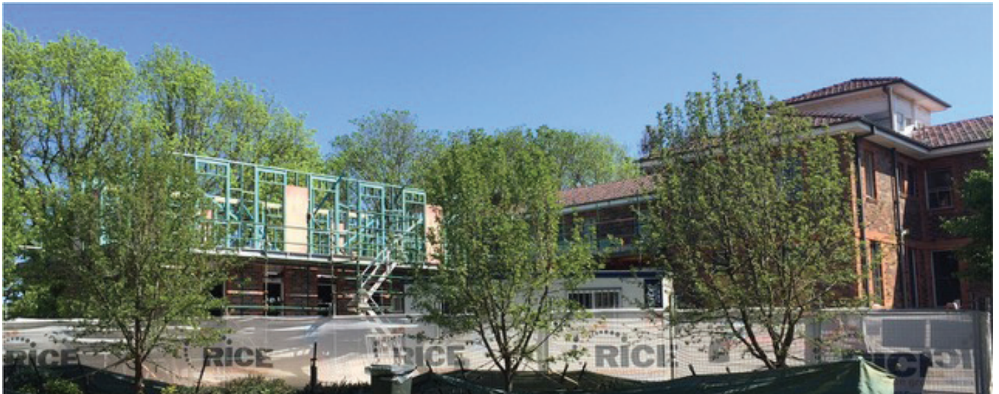
The Deakin Wing, White House, under construction
