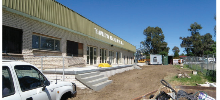
The former YCW being transformed into the Trades Training Centre
