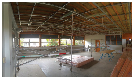
Refitting the top of Cash Building
