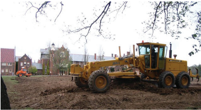
Creating the laser-levelled Adamsfield
